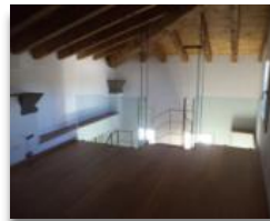
Restructuring of buildings, recovery and restoration
