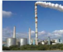
Energy establishments (cogeneration and solar)
